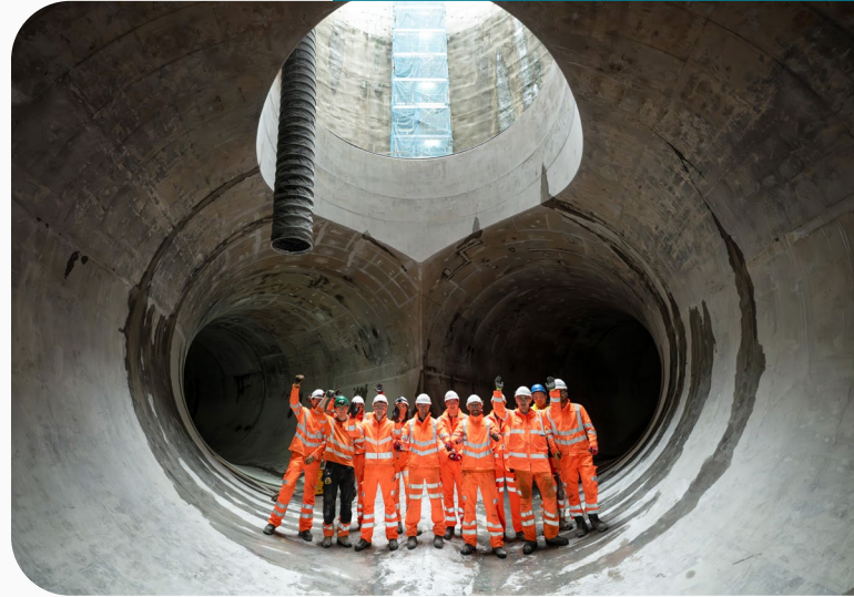
Balfour Beatty HPC Marine & Tunnels
